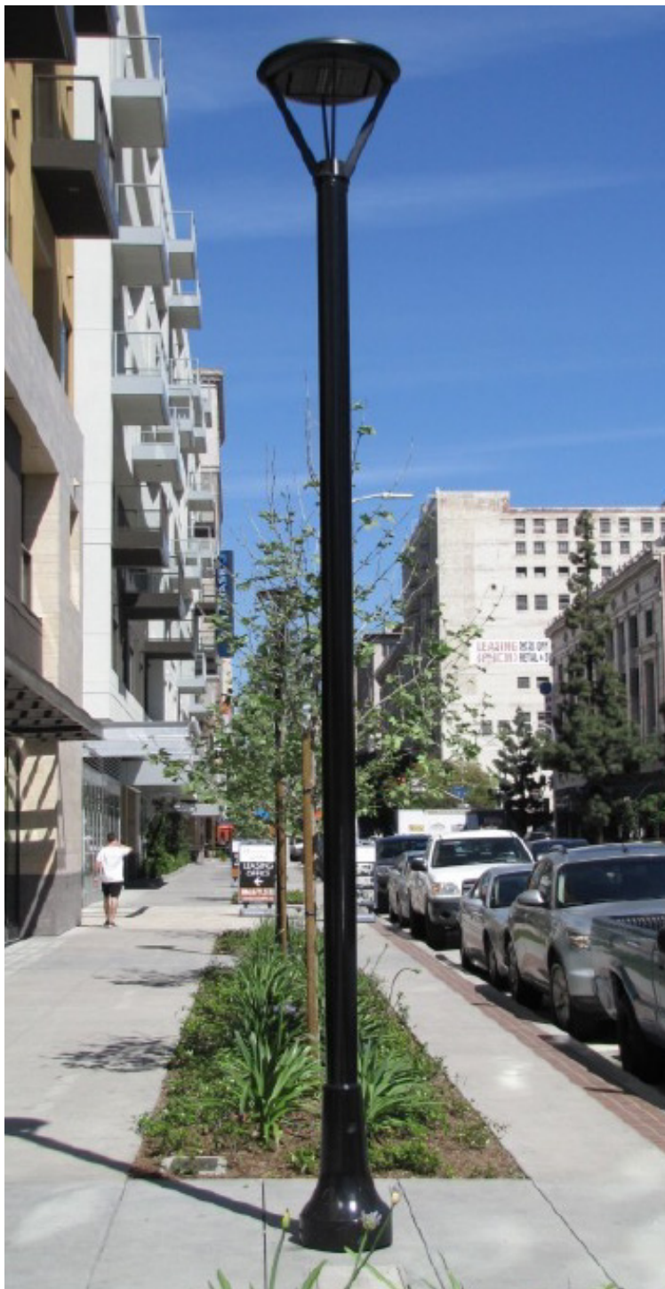
Street lighting fixture approved by Bureau of Street Lighting for use on Melrose: 14' AV Steel Pole with Cree edge round luminaire (spider)
